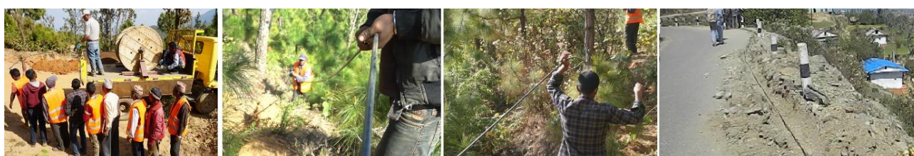
Figure 3: L.110 cable put on the ground’s surface (Jungle) and shallow buried (roadside)
